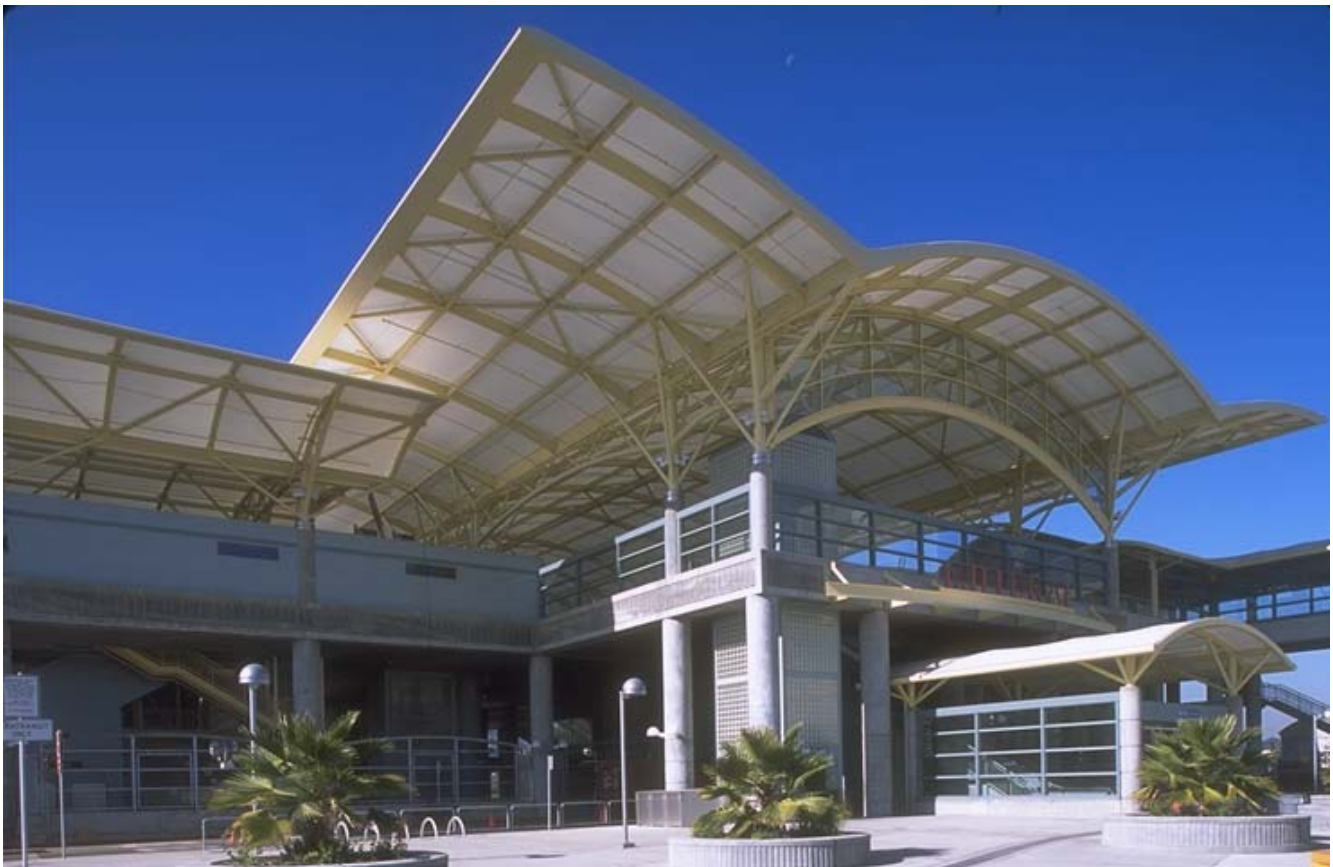
The Millbrae BART Station, part of the SFO Extension completed and put into operation in June of 2003.
