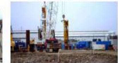
Piling - MSL Bridge over Portman Road Lane
