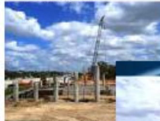
Piling @ MSL Cavern
