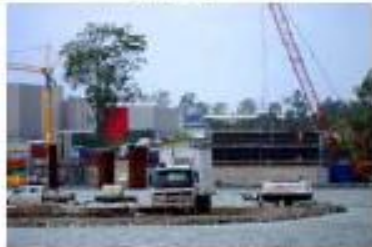
Pier 7 & 8 High Ties and Pier 9 on Barrage wall
