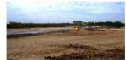
Earthworks - Zone 4 (Kippin Land)
